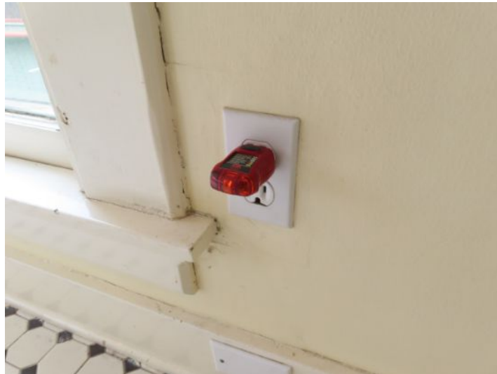
some 3 prong outlets are not grounded
