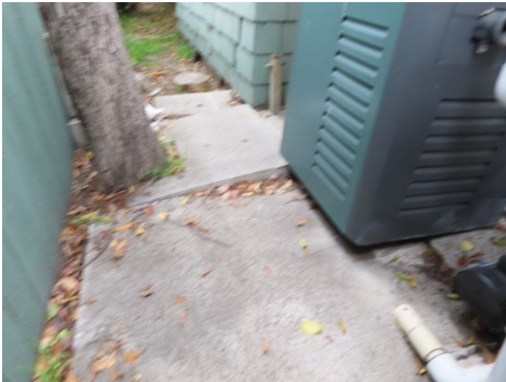
cracked and lifting concrete walkway
