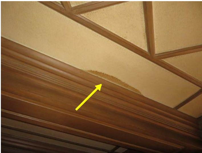
stains present, evidence of past leaking
