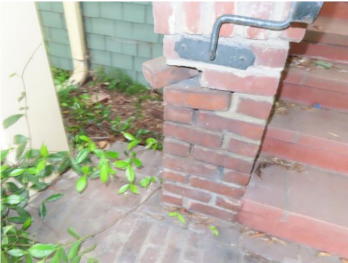
damaged and loos bricks at the porches
