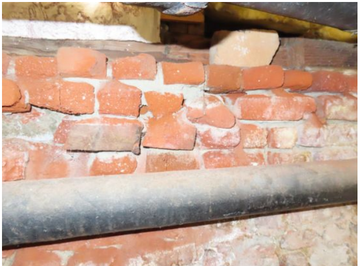
deteriorated mortar
