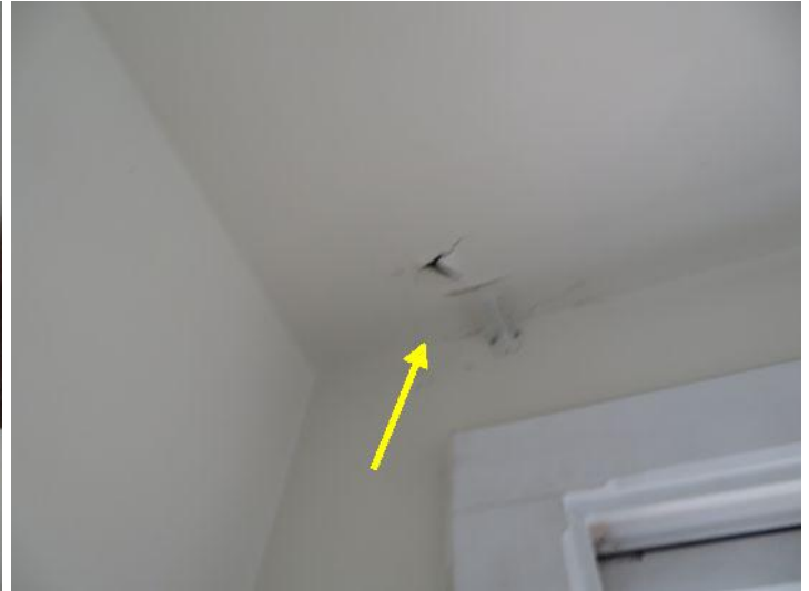
stains present, evidence of past leaking at living room
