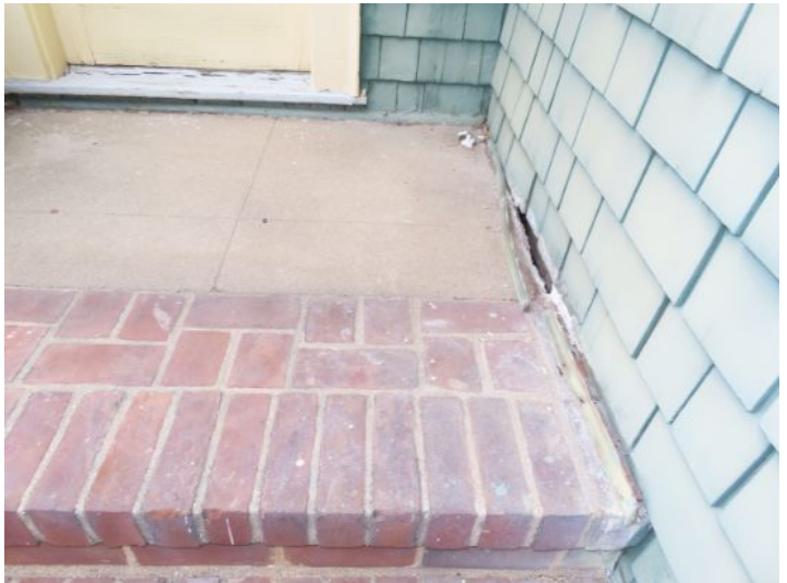
chipped, cracked and settling decks at the front porch
