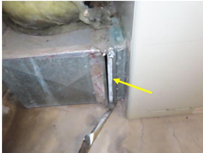
some filter access covers are missing
