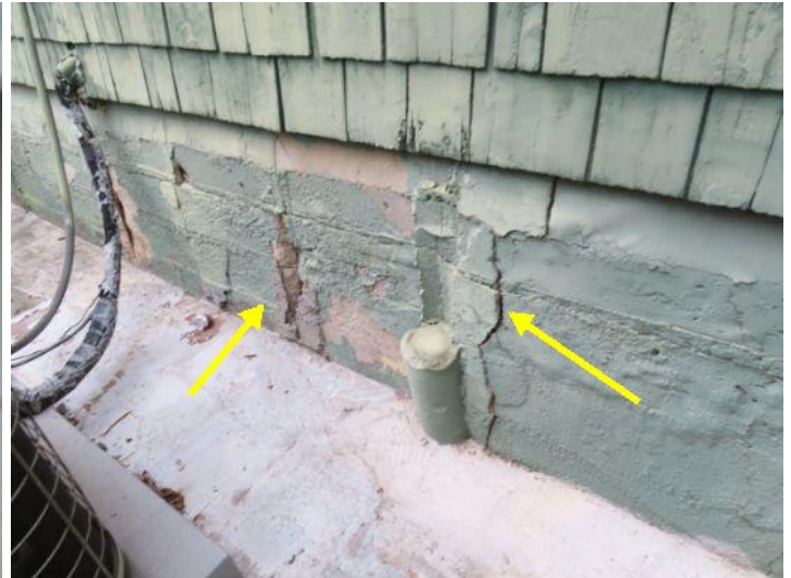
separation cracks
