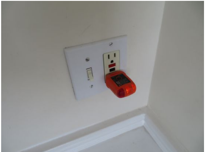
GFCI outlet present, test did not operate
