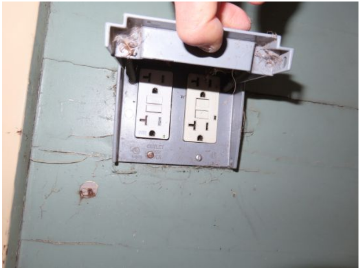
GFCI outlet has no power at the front porch
