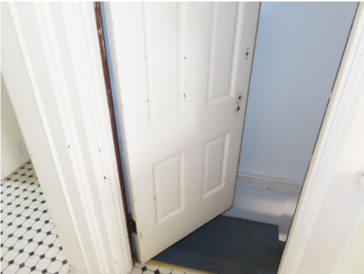
foundation access doors are broken and missing hardware
