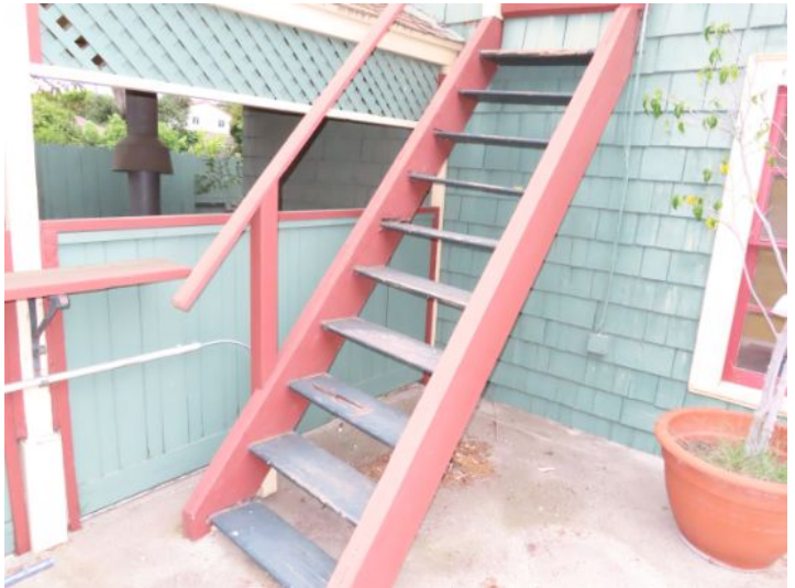
weak, damaged and deteriorated wood
