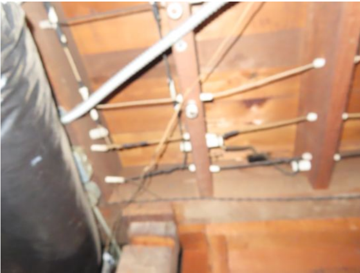
recommend upgrading knob & tub wiring
