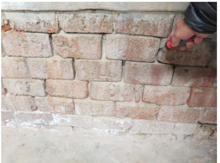
deteriorated mortar
