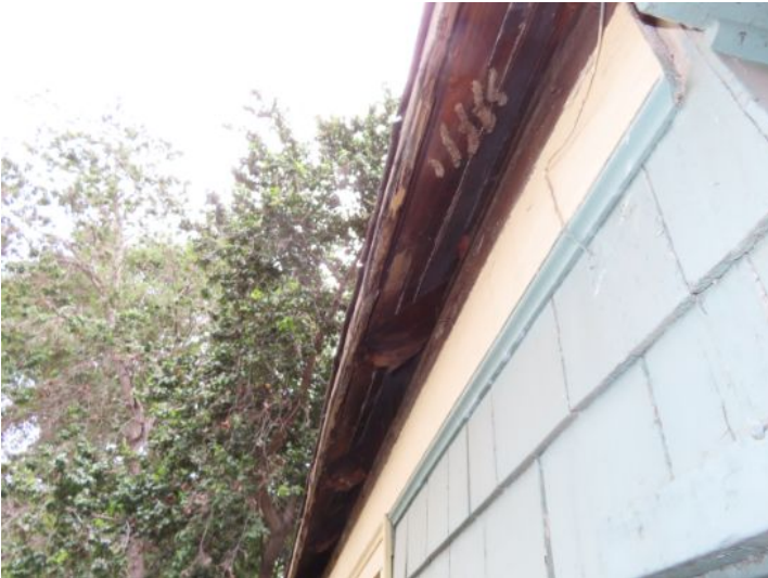
missing and loose fascia boards in areas
