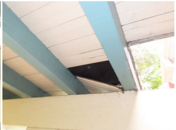
damage and deteriorated wood at all patio roof and exterior covers
