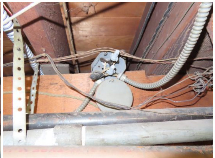
missing junction box cover
