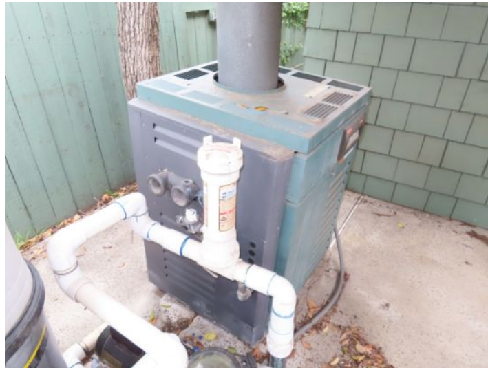
pool and spa heater did not operate, not connected
