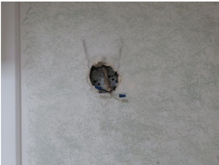
missing light fixture
