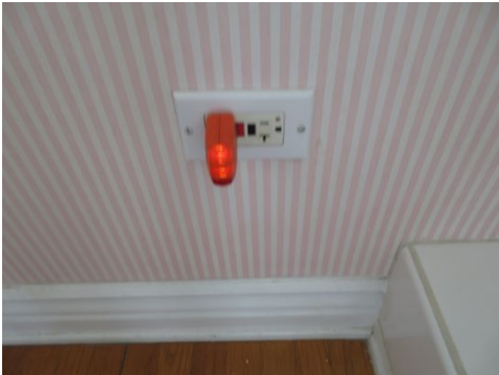
GFCI outlet present, test did not operate
