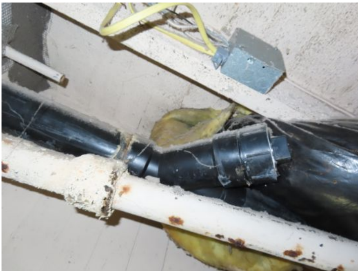
rusted and corroded, sewer drain line shows signs of leaking
