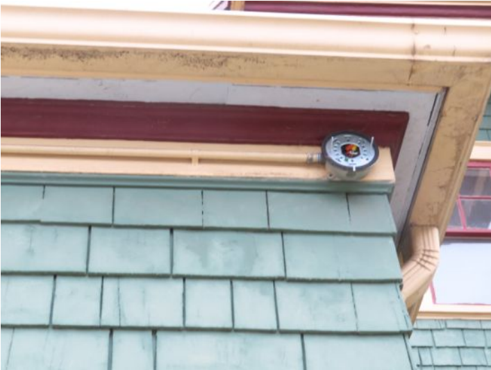
missing light fixture
