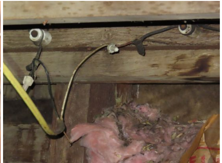
exposed connections
