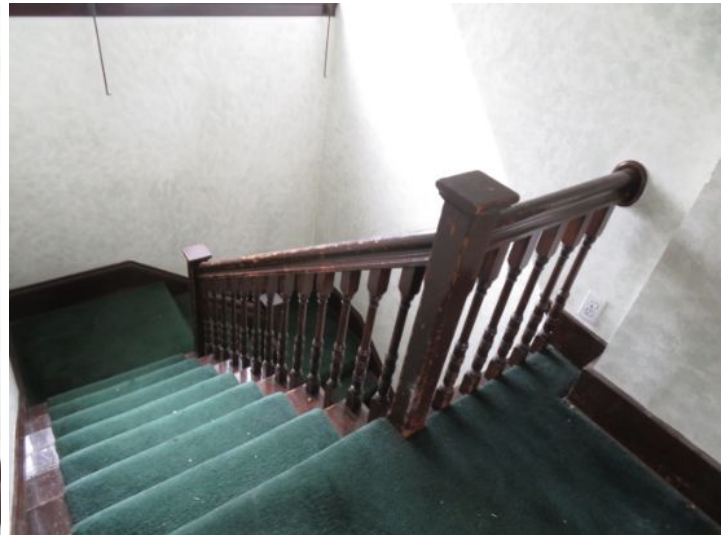
handrails are not at the proper height
