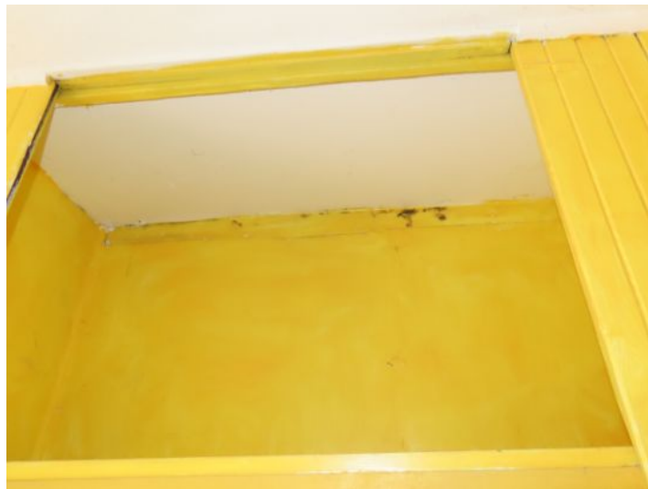
water damage and mold stains present
