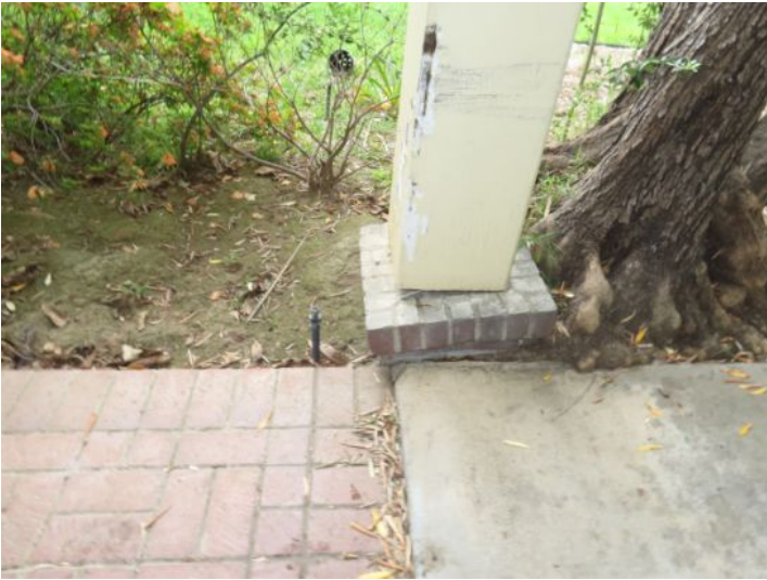
tree is damaging the support post
