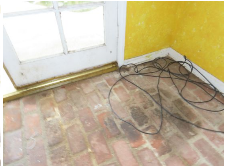
evidence of moisture entering structure
