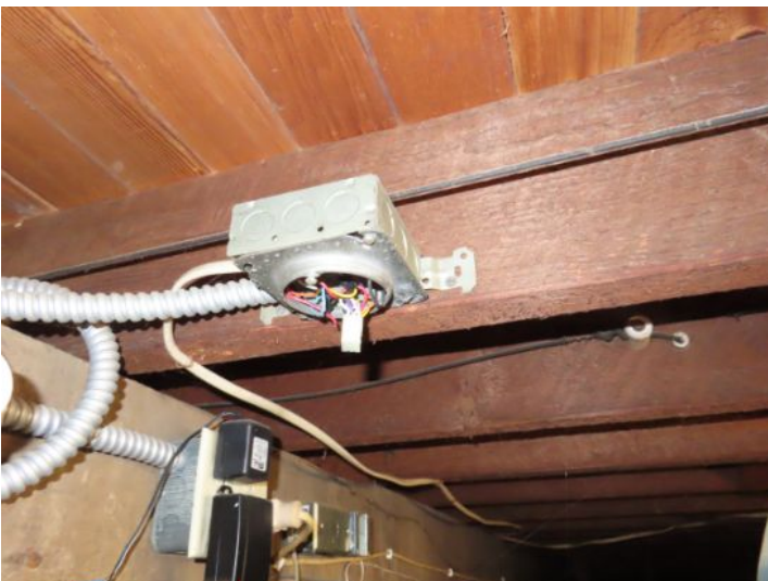
missing junction box cover
