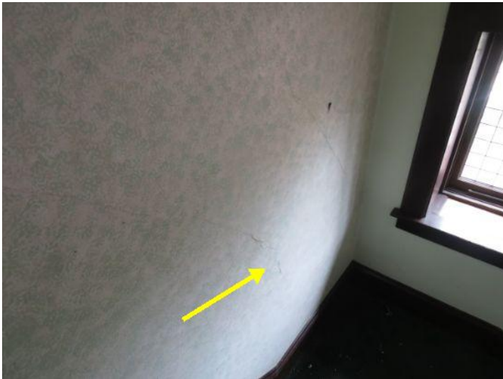
large cracks present, evidence of structural movement and shifting
