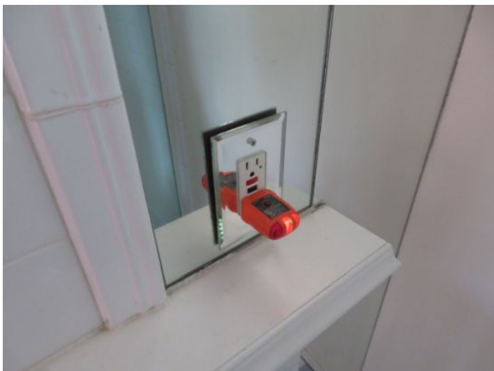
GFCI outlet is not grounded, test did not operate
