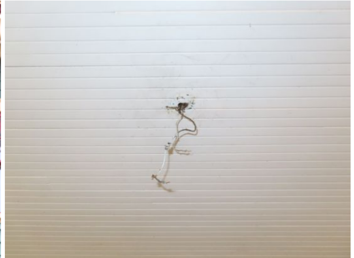
exposed wires
