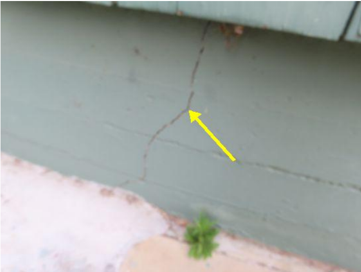
separation cracks
