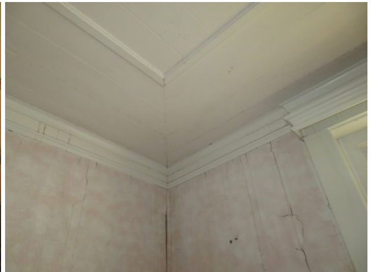
stains present, evidence of past leaking
