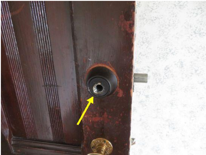
dead bolt has been drilled out
