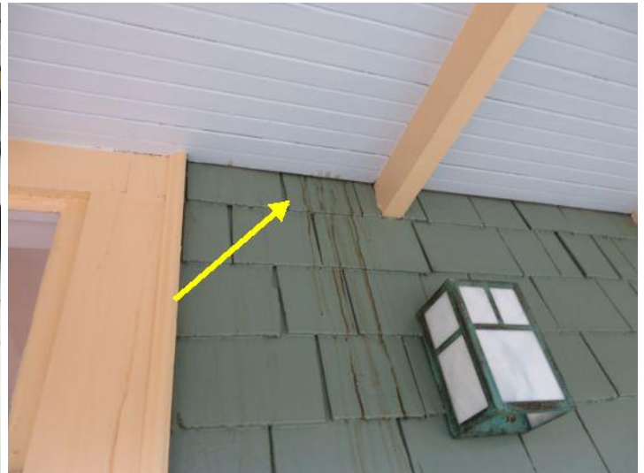
evidence of leaking at balcony roof
