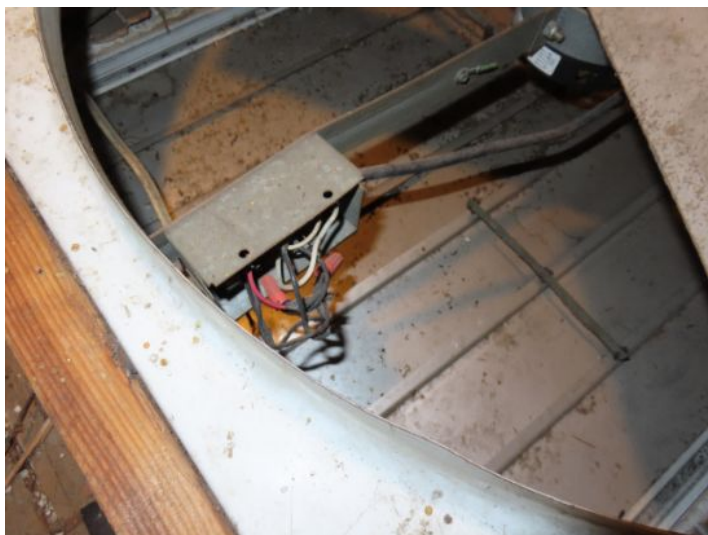
exposed wires and connections
