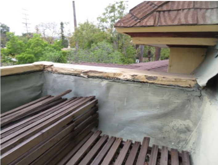
deteriorated and warped wood
