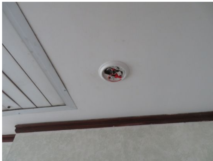
missing hard wired smoke detector
