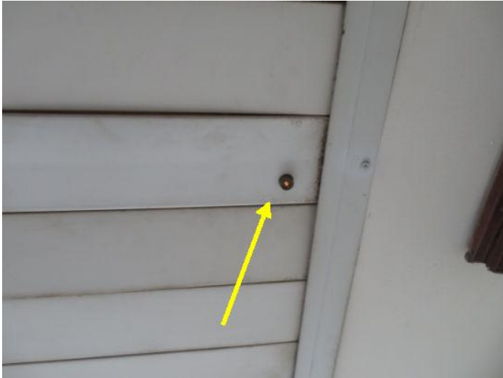
missing pull chain for whole house fan
