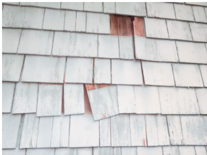
loose at the structure
