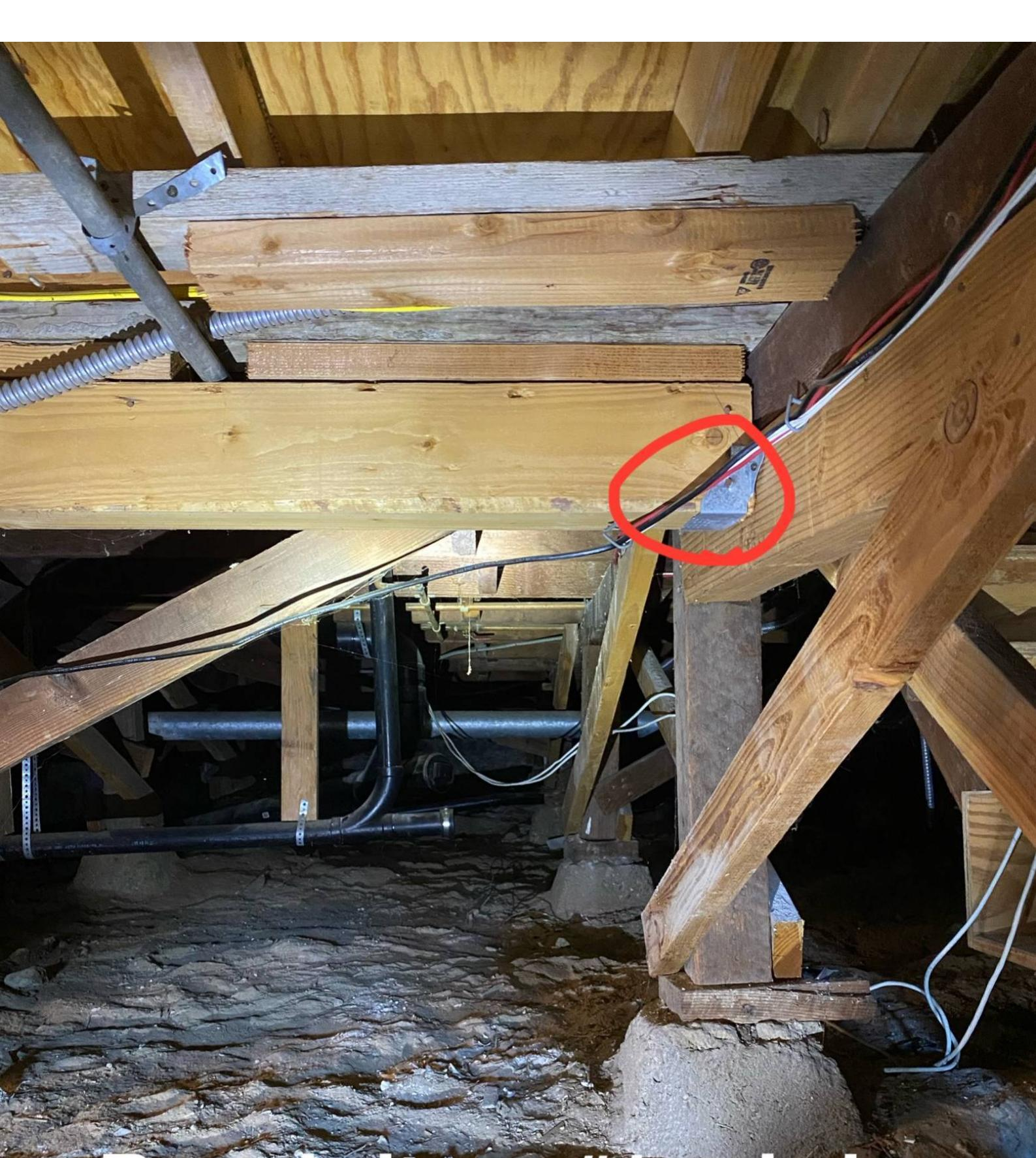
**Repair item #1: girder beams lacking adequate support**
